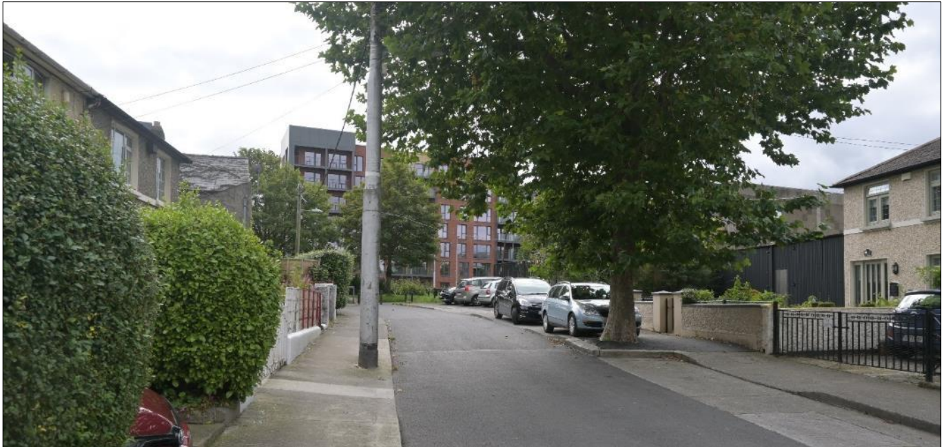
Figure 9.35 – A view from Connolly Avenue showing a new apartment development on the south side of the Grand Canal beside Goldenbridge Luas stop
