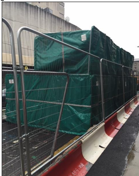
Double height acoustic blanket enclosure
