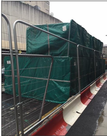
Double height acoustic blanket enclosure
