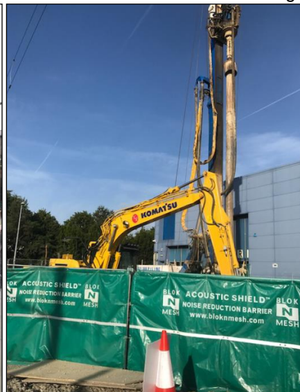
Acoustic blankets screening excavations
