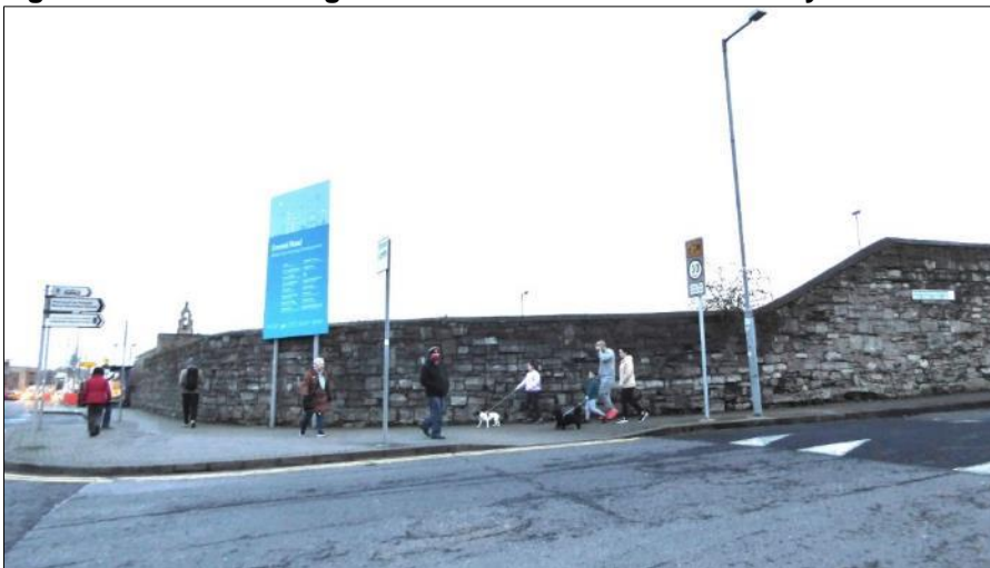
Figure 14.9 – Remaining section of the Barracks boundary wall at the northwest corner of the site
