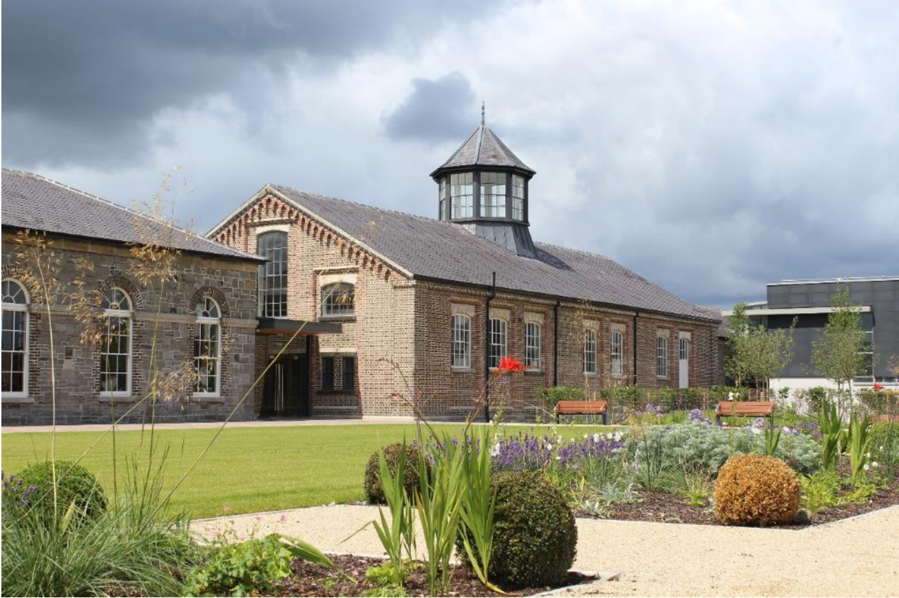
Figure 14.8 – Image taken 2106 of the eastern elevation of Gymnasium building
