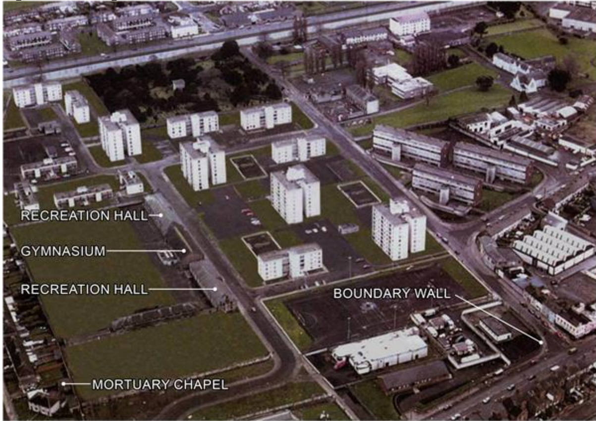
Figure 14.6 – Image taken over the site of the former barracks c.1980
