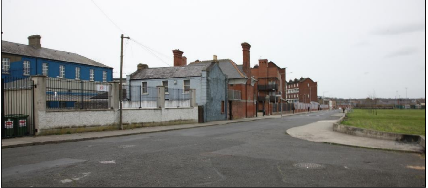
Figure 9.8 – The frontage to St Vincent Street West, with the site to the right
