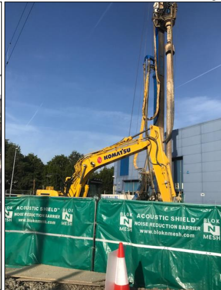
Acoustic blankets screening excavations
