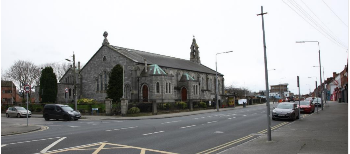
Figure 9.17 – St Michael’s Church alongside the site on Emmet Road
