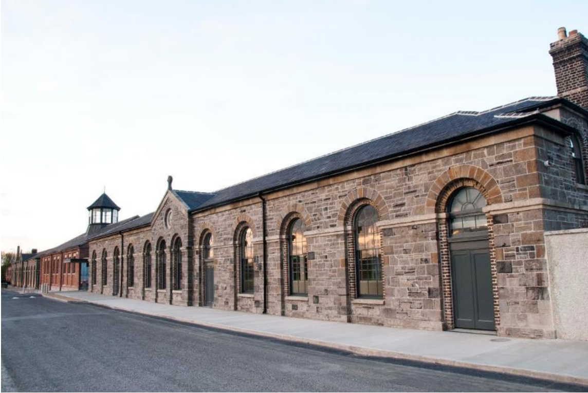
Figure 14.7 – Image taken of the western elevation of Gymnasium building in 2016
